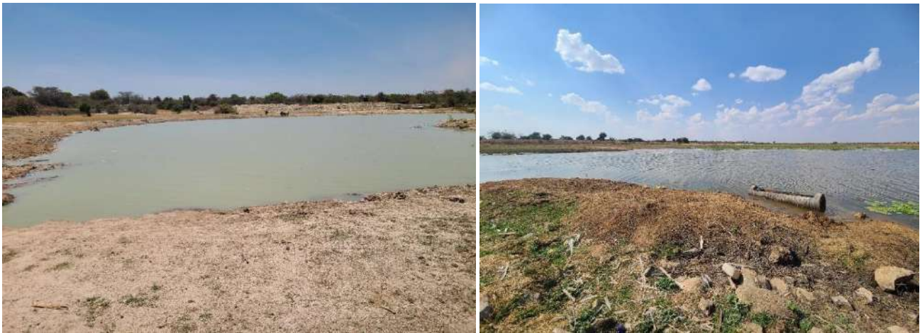
Plate 2-5: Part of Iboko dam at Utwigu Village, (2024)
