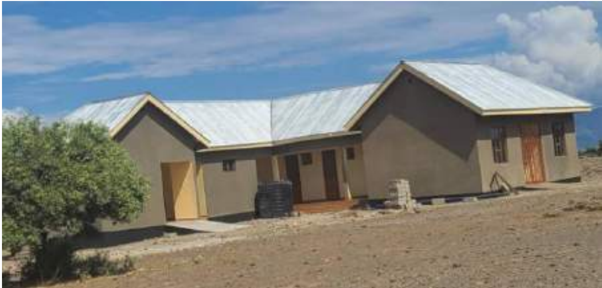
Plate 4.8: Completed Wosiwosi Dispensary Building (Not Operational)
