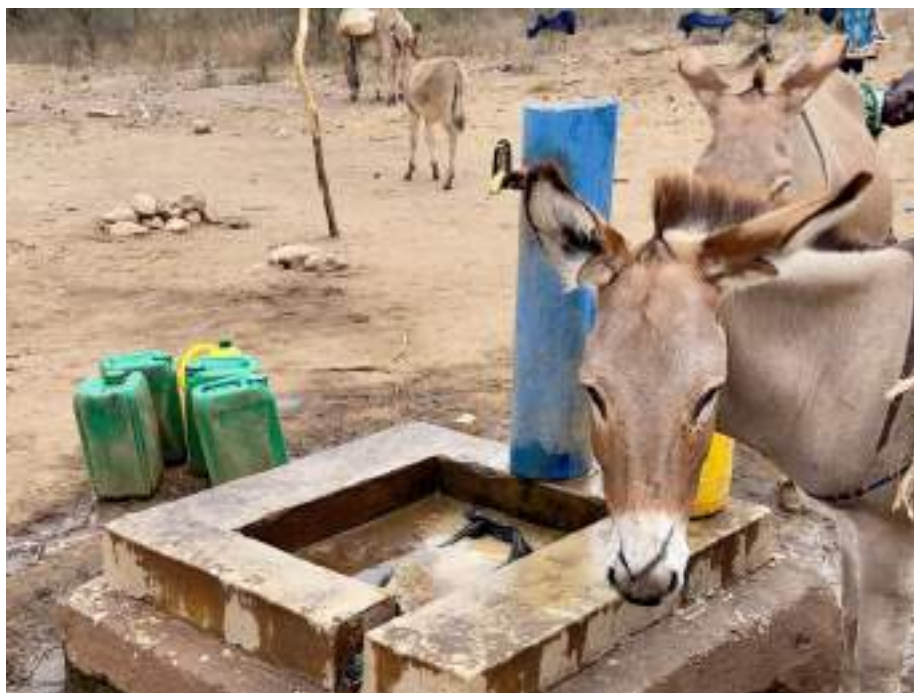
Plate 4.9: Community Water Tap in Matale B Village
