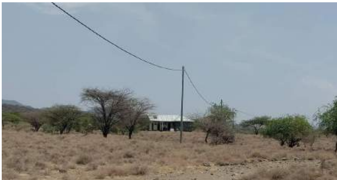
Plate 4.11: Electricity Supply in Magadini Village
